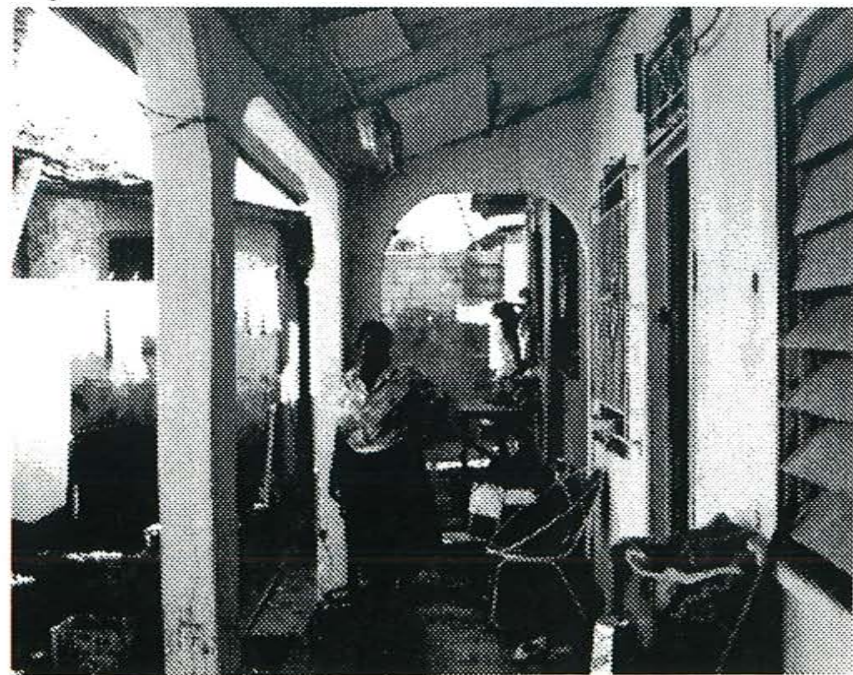
Housing in Southside: Deterioration is widespread, but the housing is livable in the benign climate.
